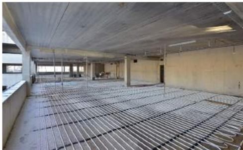
Water-filled coils running through the "active" floors, 15 cm apart, giving 4.5 m of pipes/m<sup>2</sup>
