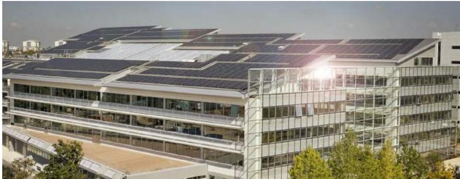
30% of the hot water requirement is produced by solar panels.
