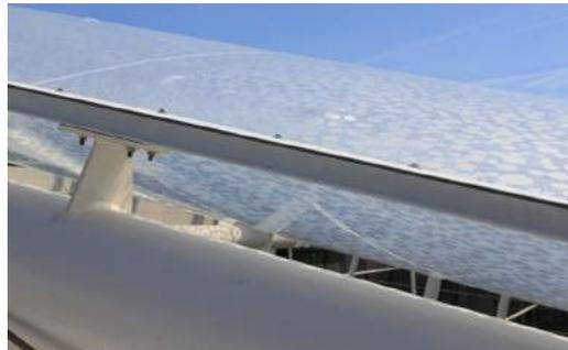
This has enabled a low consumption covered space to be created. In winter, a slight warming reduces the need from the internal facades of the garden. In summer, convection creates a cooling draught, eliminating naturally any greenhouse effect.
